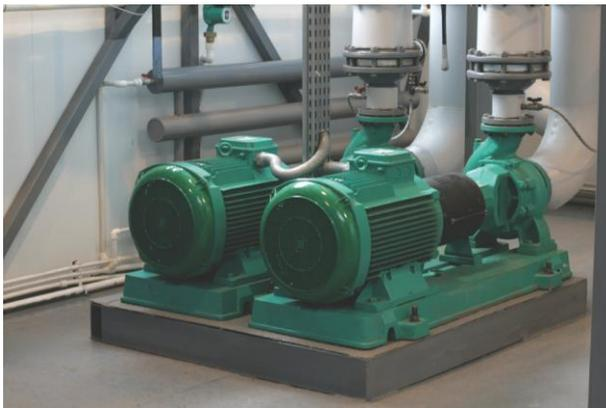
*Pump Control – Water/wastewater system pump controls is typically a relatively simple application that can easily be handled by a smart inverter.*
