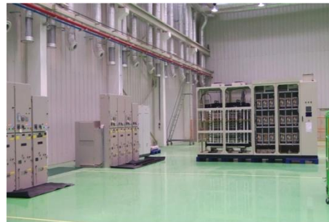
6.6 kV Drive Under Test
