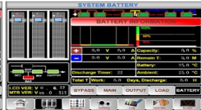
(a) Interface of Battery
