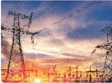
Power Generation & Utility Industries
