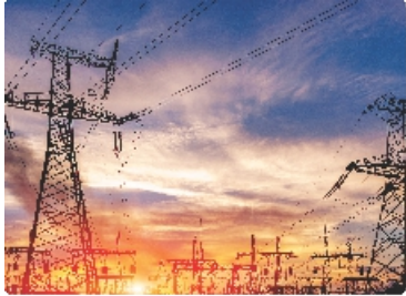
Power Generation & Utility Industries
