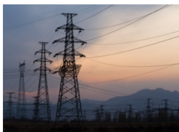
Power Generation & Utility Industries
